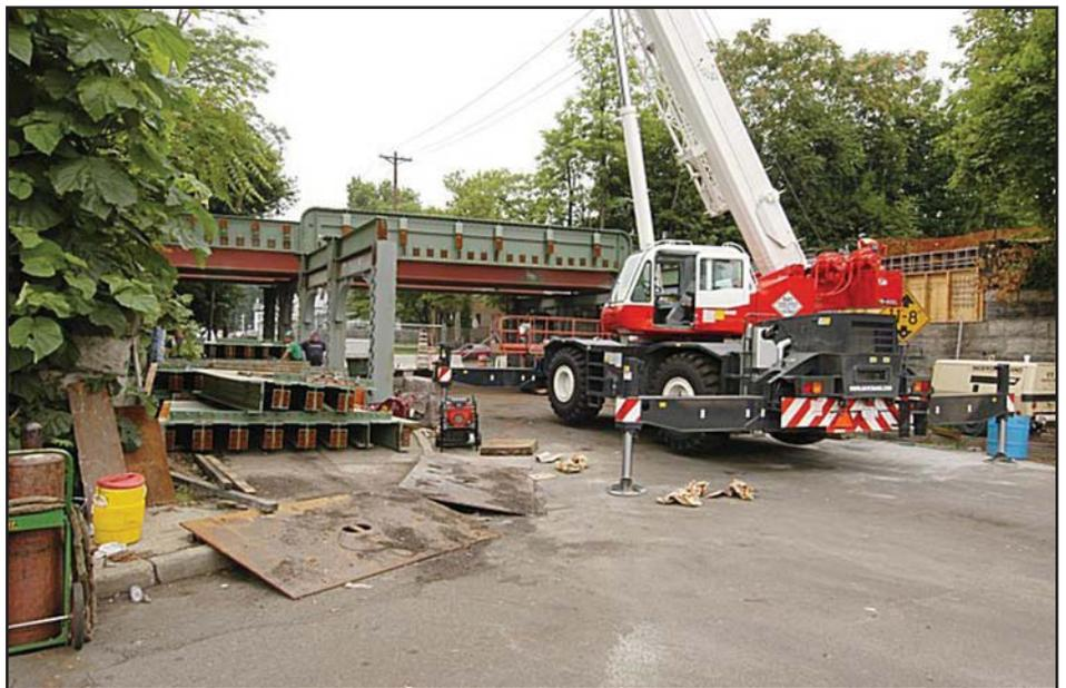
**Steel erection for the NJ Transit bridge rehab in Plainfield. Final work required intensive historic replication.**
